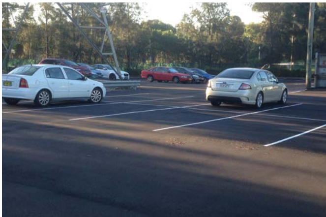
The resurfacing works are now complete.
