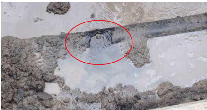
Domestic water cast iron pipe burst section
