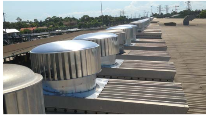
Smoke Evacuation Vents fitted to Building 'E' Roof
