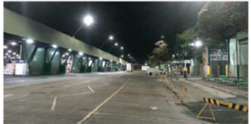
South Road Lighting
