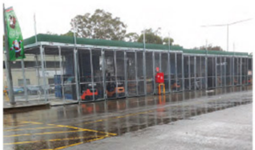
Completed Forklift Enclosures
