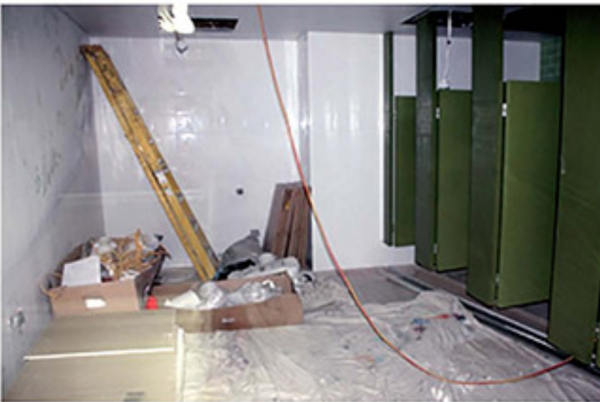
L1 amenities almost complete
