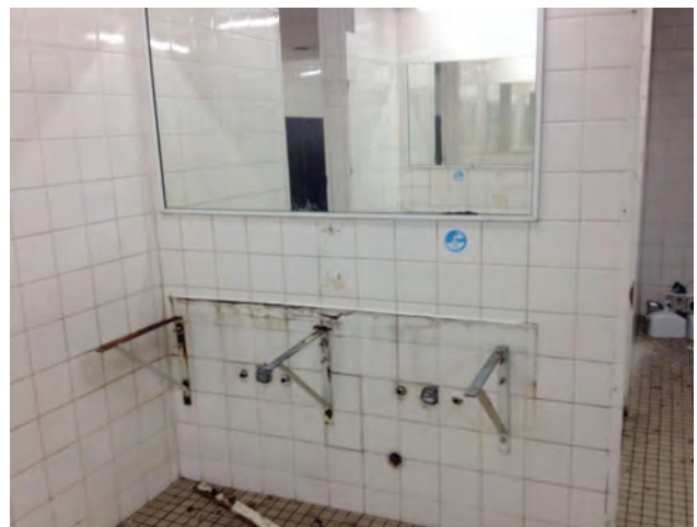
Demolition works inside the amenity area
