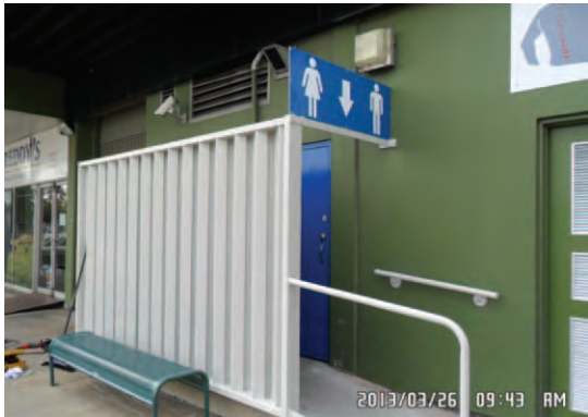
New Public Toilet on western side of Plaza
