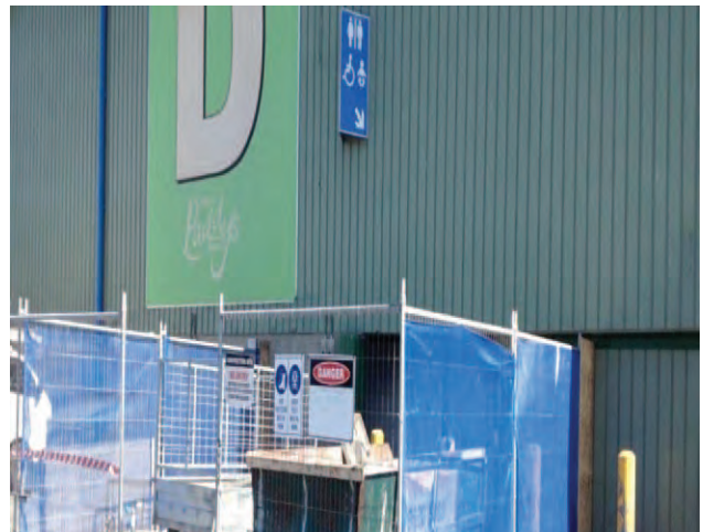
Storage area for builder on the eastern side of Building 'D'
