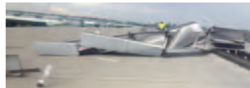
Roof Ridge Vent torn off on Building 'G'
