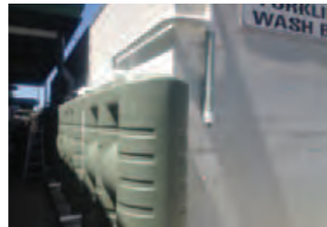
Water harvesting tanks installed to supply water for forklift wash down
