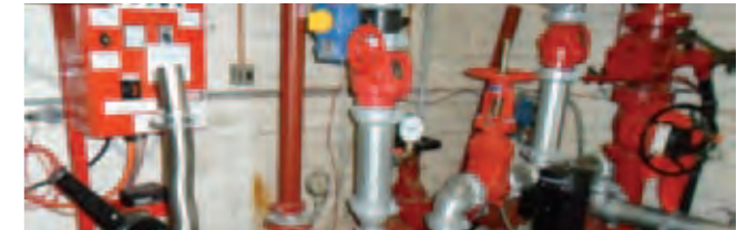
New hydrant pump set up adjacent to the existing sprinkler pump
