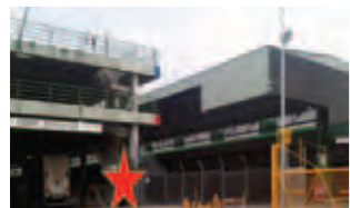
Car Park Lift Location
