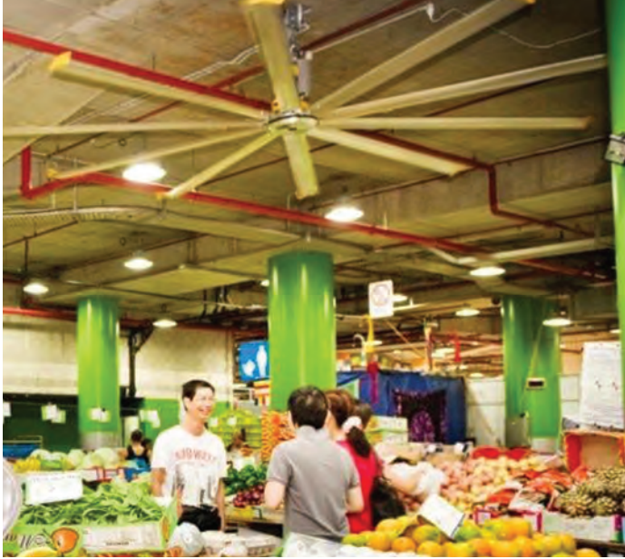
New fans and lights recently installed at Haymarket.
