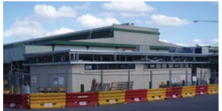
Sydney Markets Credit Service under construction
