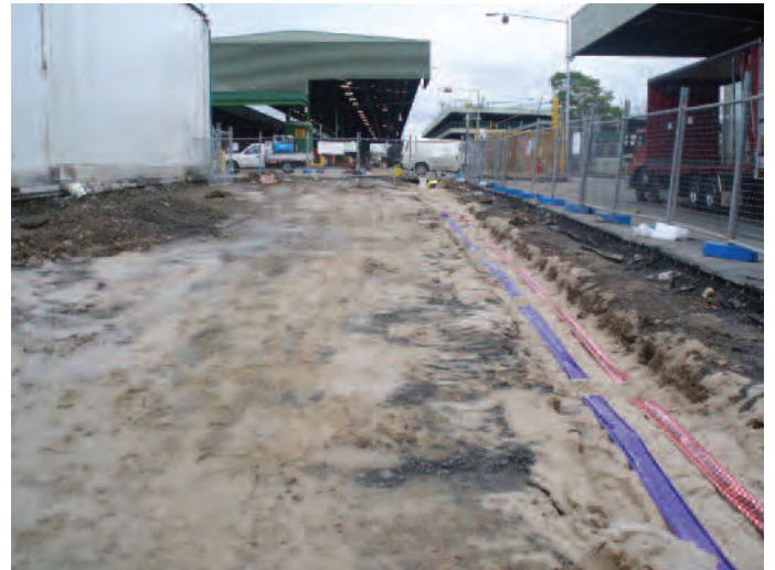
Preparation of ground prior to regrading.
