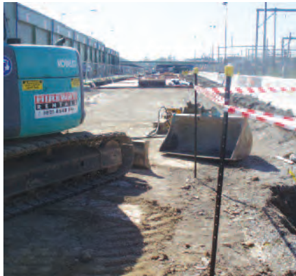
Excavation works completed.
