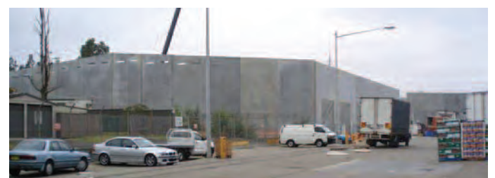
Erection of concrete wall panels.
